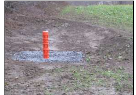
This water and sediment control basin (WASCOB) with a 6" standpipe and tile outlet was installed with the ACRF funds to prevent erosion due to surface water flows from the upslope drainage area.
