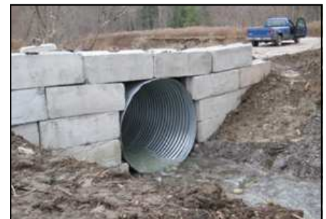
An 8 foot culvert was used to handle the flows of this stream. An earthen spillway was also excavated in the crossing to serve as an area for flood water to escape if a blockage ever occurred in the pipe. Concrete waste blocks were used for the headwalls.
