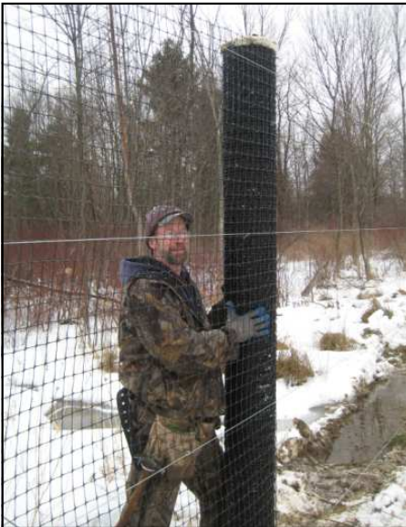
Madison County’s Jerry Boyd building deer fence.
