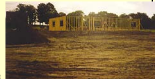
Outside shell installed
