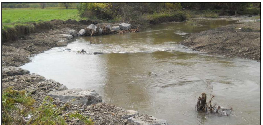
Rock across the stream creating a riffle and protecting the farm field.
