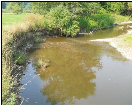
Erosion along the stream banks resulting in the loss of land.
