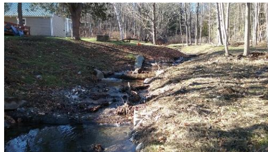
December 2017, 2 months post-construction; upstream view; log and rock grade control structures stabilize the bed and provide habitat.
