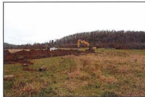
WASCOB outlet repair in November 2016 which included resizing the pipe and re-grading the spillway.
