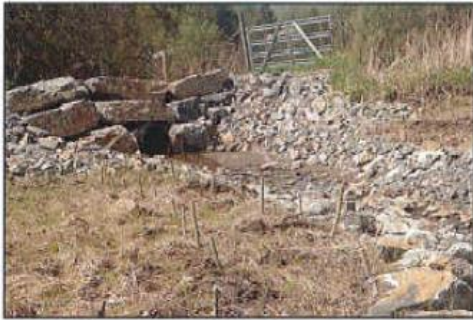
AEM Tier 4 Access Road and Culvert Crossing Project completed October 2015 – with willow plantings for channel stabilization in April of 2016
