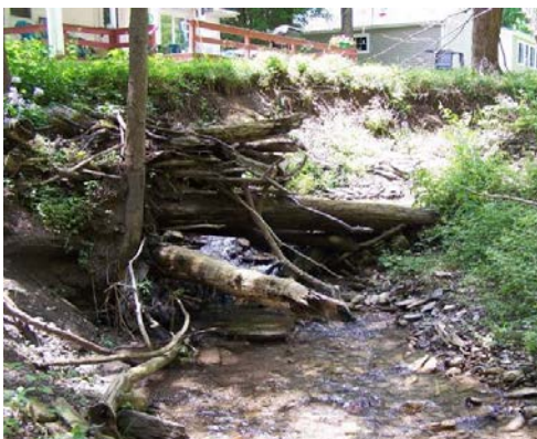
Upstream View: June 2016, erosive bank, debris blocking channel, incised conditions.
