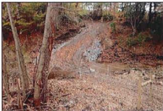
This stream crossing and cattle lane was installed in October 2016 to protect the water quality of a blue line stream
