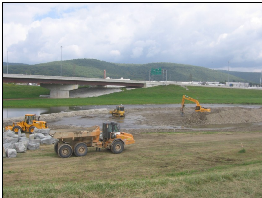
Gravel Deposition Removal Used on the Eroding Bank
