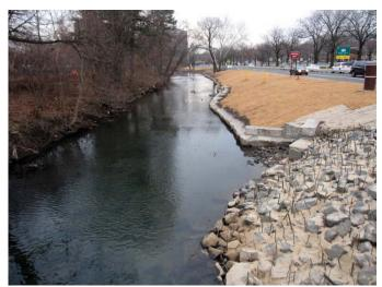
installed riparian buffer plantings towards stream protection and wildlife enhancementand also recognized the needs of disabled individuals through installation of permeable pavers facilitating stream access with cantilever sampling decks.
