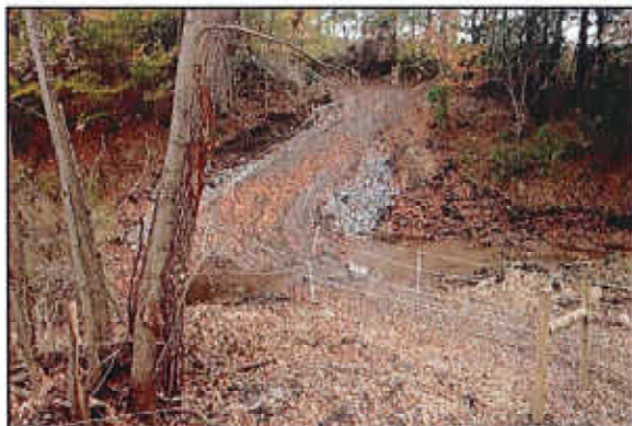
This stream crossing and cattle lane was installed in October 2016 to protect the water quality of a blue line stream
