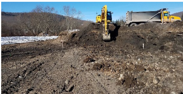
Photo shows the depth of material excavated from the project. The material was sorted prior to off-site trucking to remove debris and solid waste.
