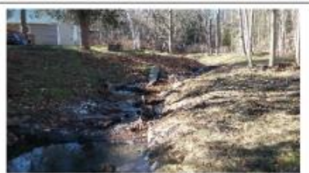
December 2017, 2 months post-construction; upstream view; log and rock grade control structures stabilize the bed and provide habitat.
