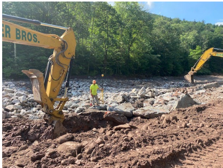
Installation of boulder revetment for stream bank stabilization.
