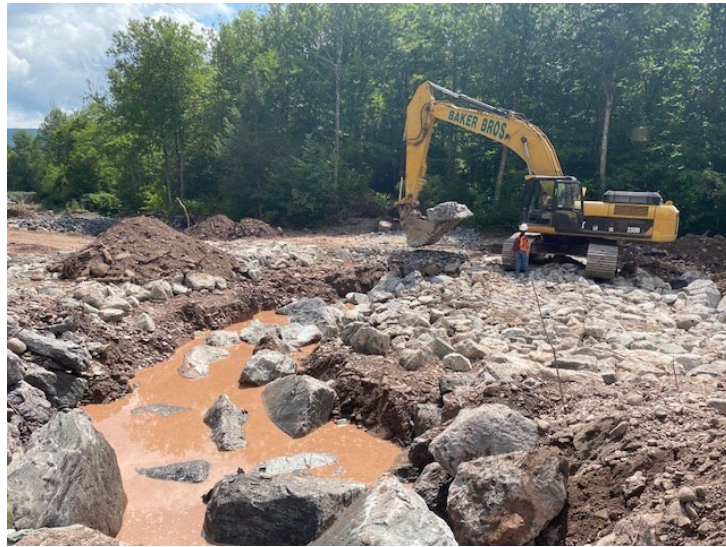
Installation of boulder riffle structure for stream grade control.
