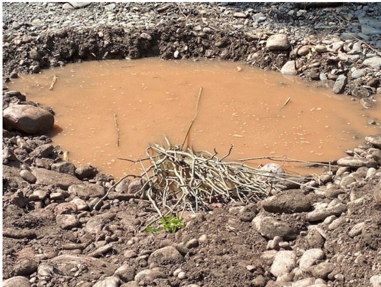
Soaked willows for installation in boulder revetment. Vegetation is an important component of streambank stabilization. The installed willows are watered on a daily basis.
