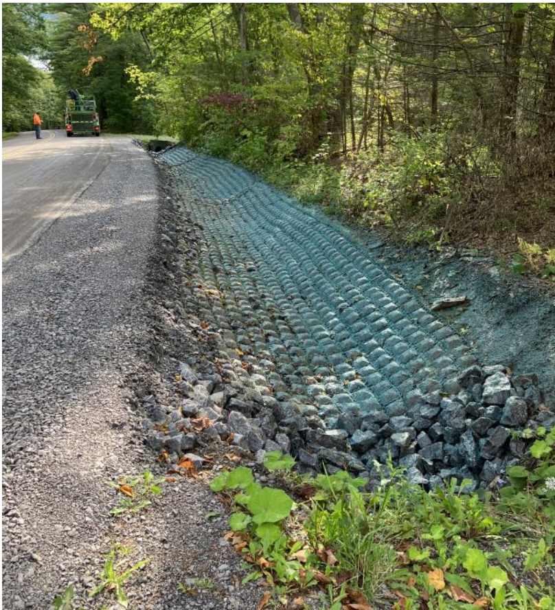
This is Flexamat material being installed along a steep roadside ditch leading to Honeoye Lake. The Town of Canadice installed the material as part of the WQIP Round 17 and the Ontario County DPW partnered to hydroseed the project upon completion. We have installed this material in several locations within the Honeoye and Canadice watersheds with a lot of success! Photo by Katie Lafler, Ontario County SWCD.
