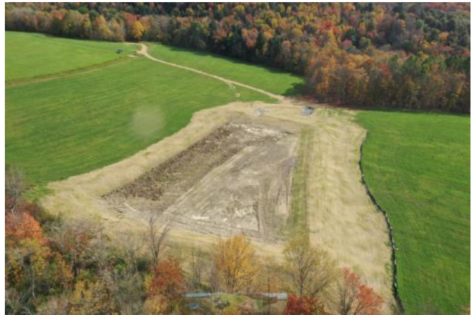
Tioga SWCD completed construction on a small retention pond project funded through CRF R6 to mitigate erosion in a sugarbush, reduce peak stormflows from the property and add resiliency to the watershed. The project will receive a riparian forest buffer planting this spring along the active cropfield as the final component.
