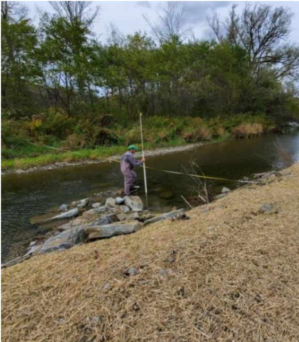
Tioga SWCD Stream Technician Mike Jura wrapping up construction on an AGNPS R28 project this fall. The project utilized riprap with rootballs, barbs and live willow plantings to stabilize the streambank. A riparian forest buffer planting will be added in the spring to finish the project.
