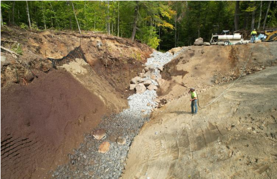
District Technician Lenny Croote hydroseeds biotic soil media and grass seed on top of Geoweb to prevent erosion at the Gilmantown Road bank stabilization project site.
