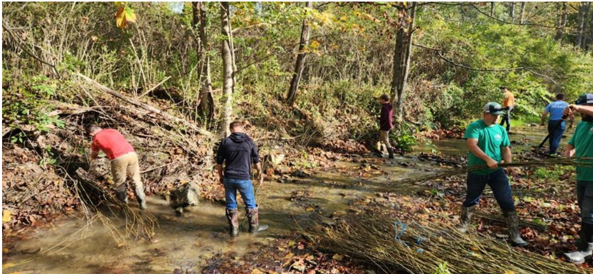
GST BOCES Students staking the prepped willow cuttings into sections of eroding stream bank.
