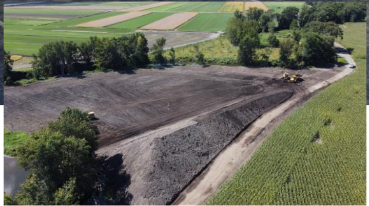
This is a drone picture, taken by one of the landowners of this Orange County SWCD project site. It shows the ongoing construction of floodplain benches/riparian forest buffers along the Wallkill River. It depicts fairly well how the bench/buffer will insulate the river from the adjacent cropland while mitigating agricultural flooding.
