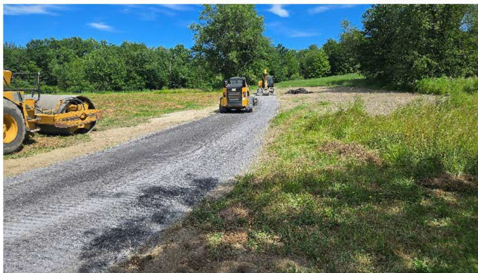
Access road in same location after improvement
