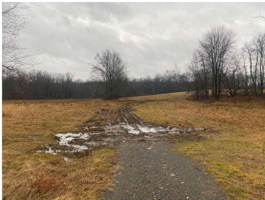
Access road before improvement
